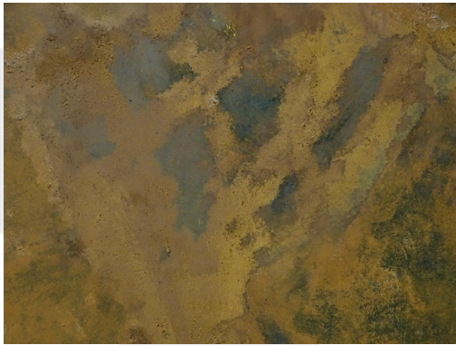
Patches of RED RUST applied with a paste of RED RUST
